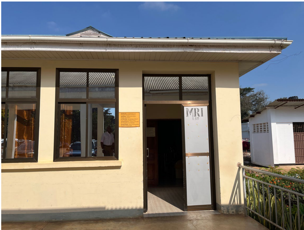
1.5 Tesla MRI housed separately from the main hospital building
